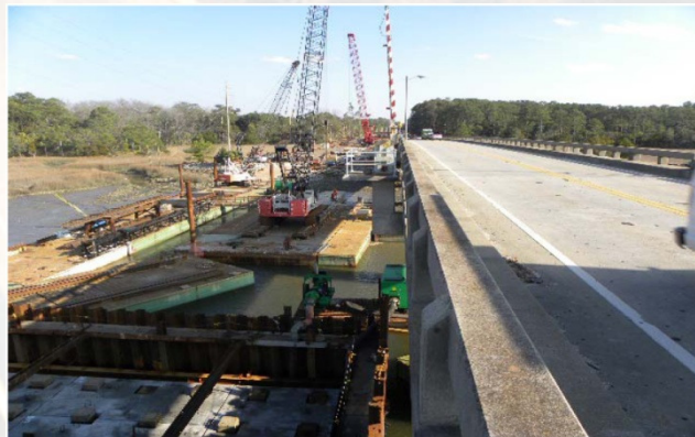
Skidaway Narrows Bridge Replacement
